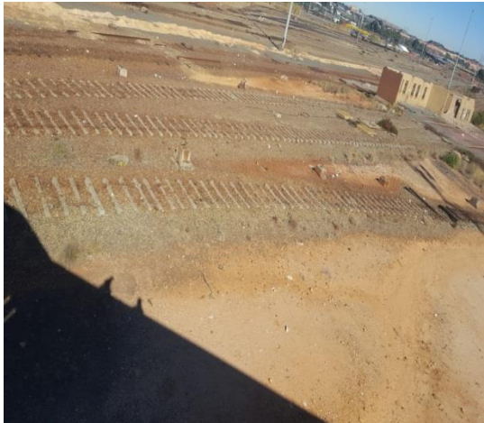
Fig 2.3: Vandalized staging yard
