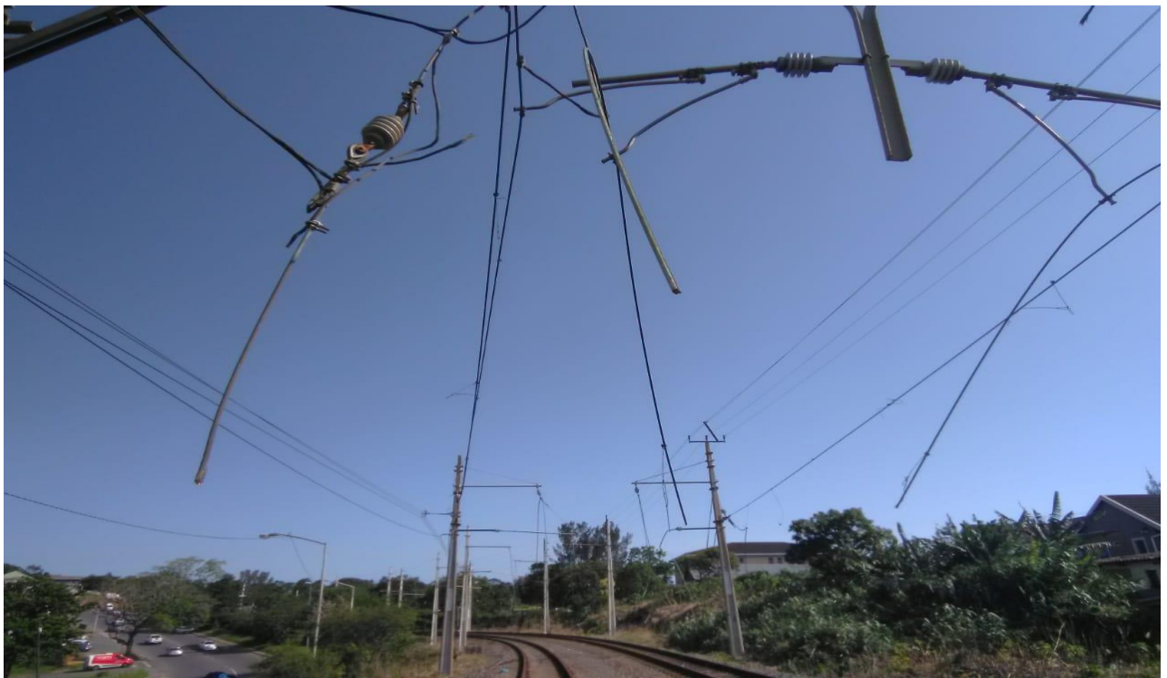
Picture 2 OHTE wires hanging low due to theft and vandalism
