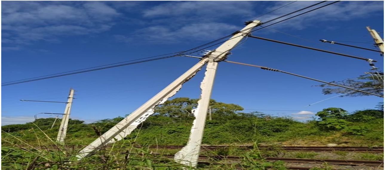
Picture1 Cracked mast pole
