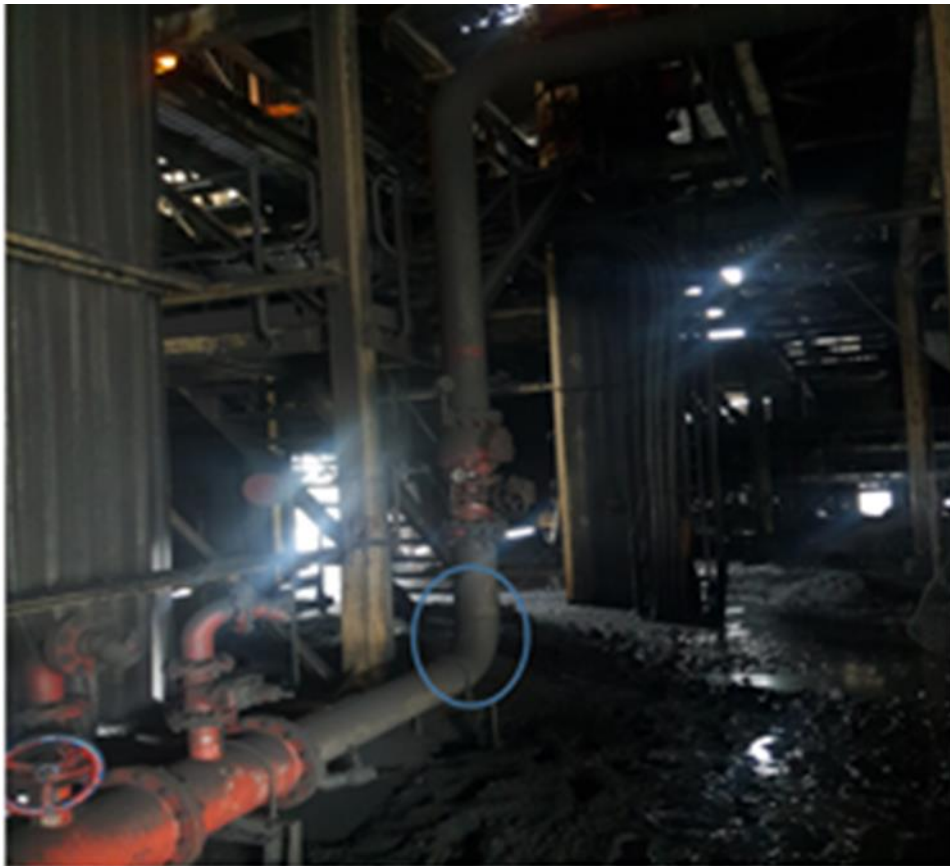
Figure 2: Existing Fire reticulation to be re-routed at Sizing Complex.
