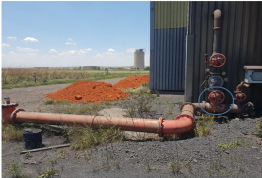
Figure 5: Existing Fire reticulation at been feeder to be demolished.
