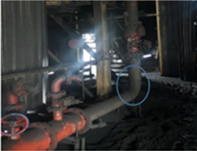
Figure 3: Existing Fire reticulation to be re-routed at Sizing Complex.
