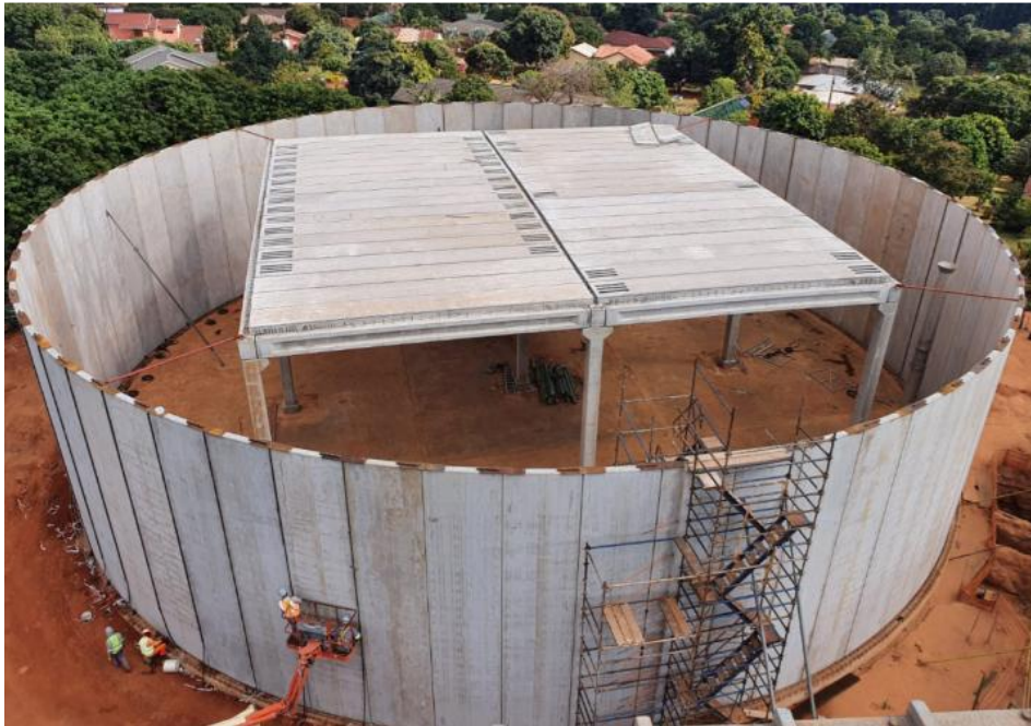
Figure 12: Typical View of Precast Walls
