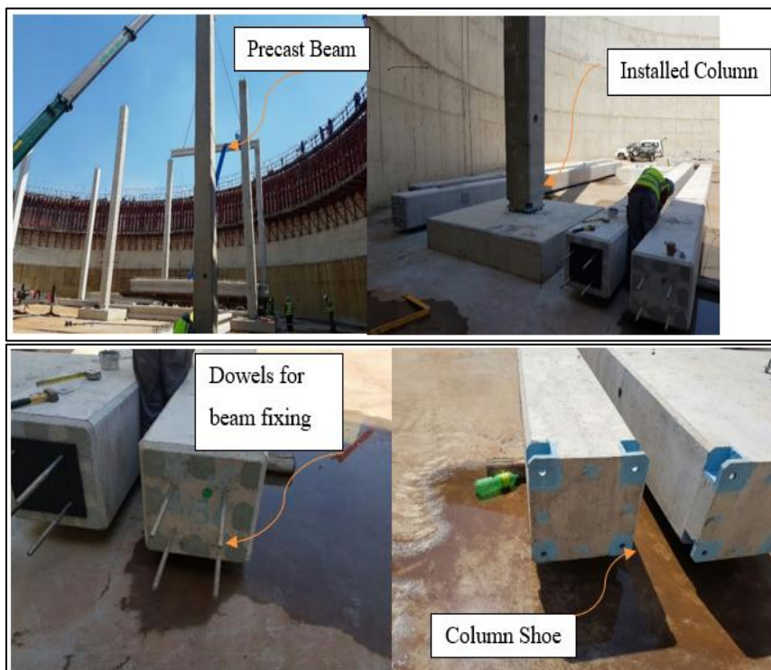
Figure 8: Typical beam-column-slab interface
