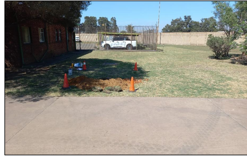
Picture 2: Looking south along the alignment of the new pipe racking and bridge, which will pass alongside the existing change rooms.
