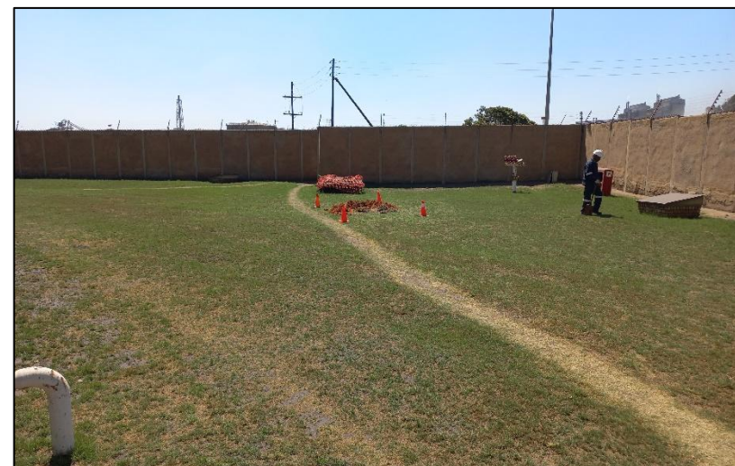
Picture 4: Looking north across the proposed valve bank which will be positioned in the north eastern corner of the site.
