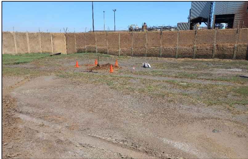
Picture 3: Looking west towards the proposed valve bank position on the western edge of the site. This area appears to suffer from frequent flooding.
