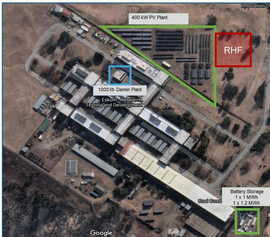
Eskom Research and Innovation Centre (ERIC) at Rosherville illustrating the RHF location.
