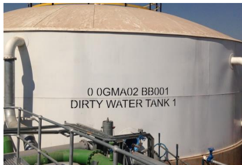
Figure 33: Round Vessels stencil example
