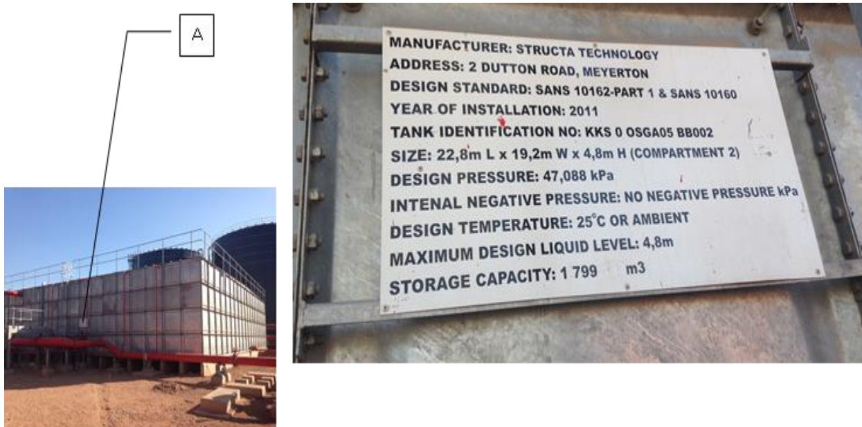
Figure 34: Square vessels Detail A
