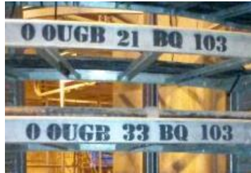
Figure 36: Cable rack/tray stencilled example
