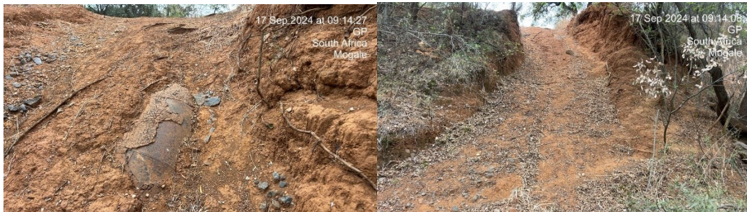
Fig1.1.1 Picture showing the exposed pipeline.
