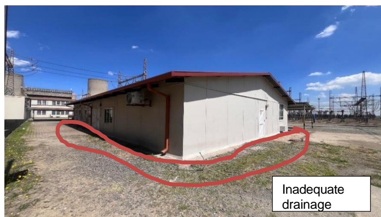
Figure 12: Existing drainage at D&S building
