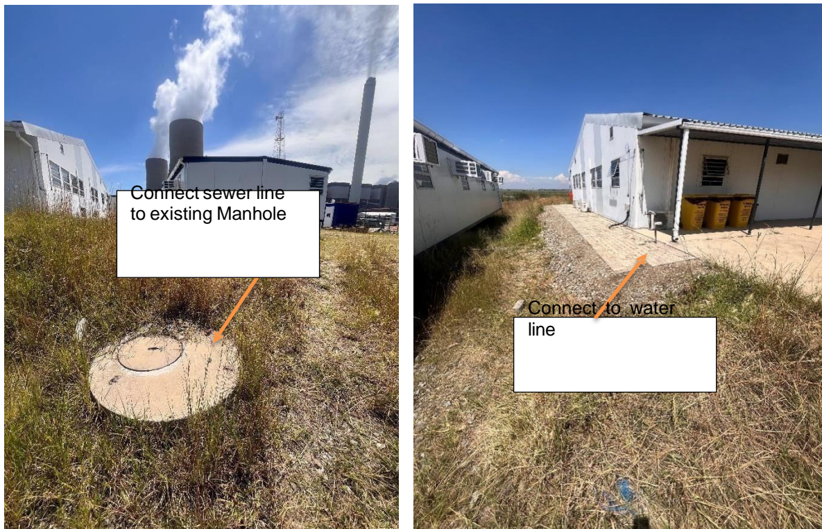
Figure 2: Proposed sewer pipe layout GCD
