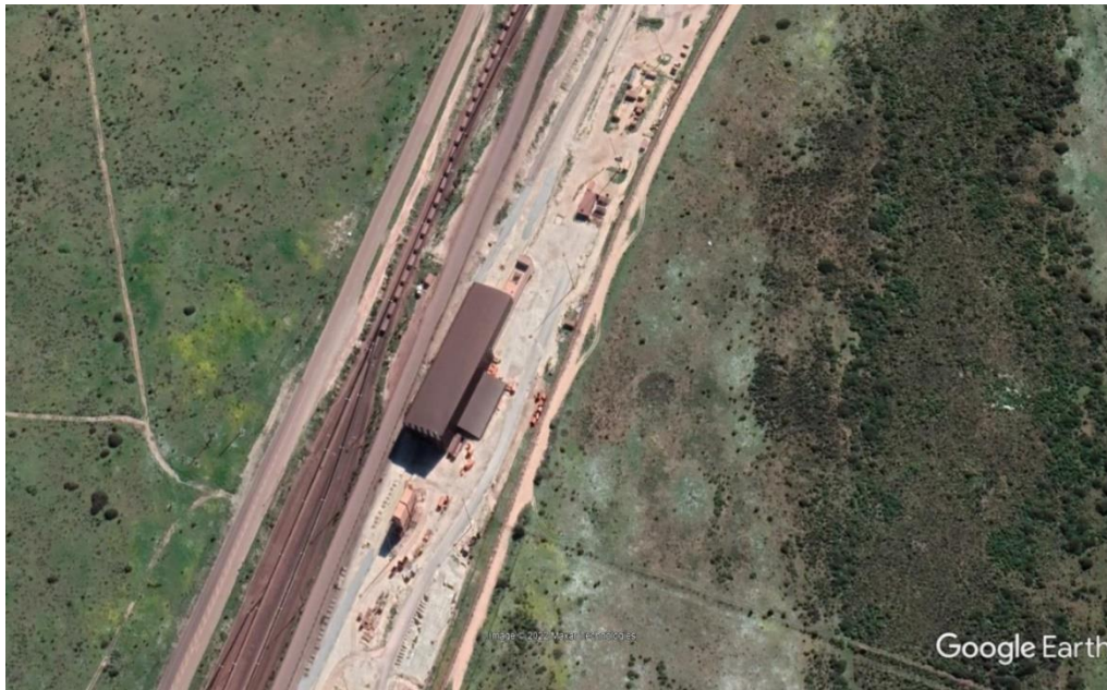
Figure 1: Aerial View of Tippler 3
