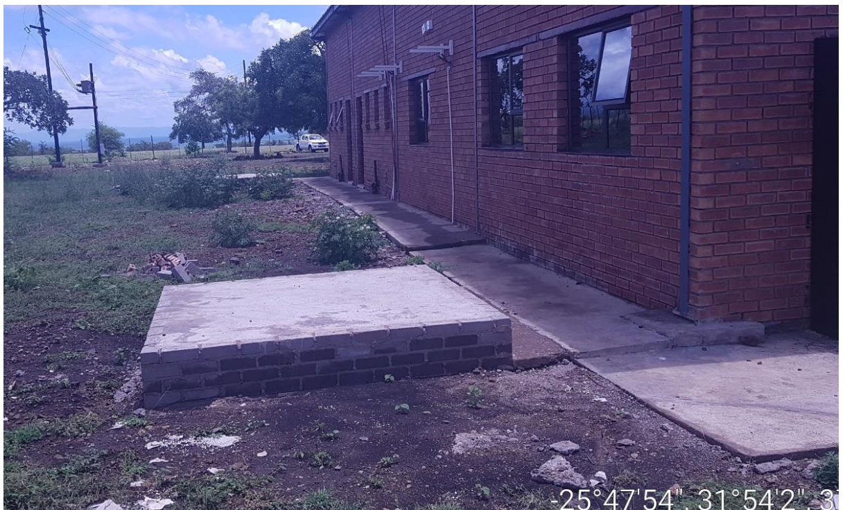
Photo: Existing platform for water tank. Room for pressure pump is in the building next to the tank
