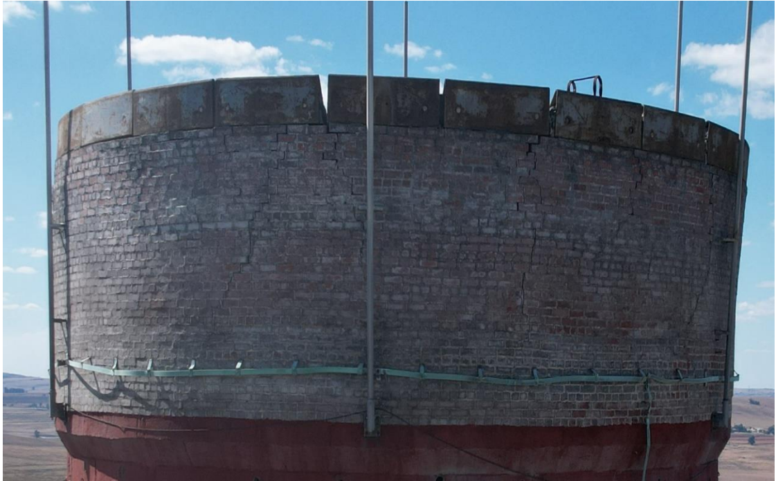
Diagonal brick wall cracks: Southern Chimney
