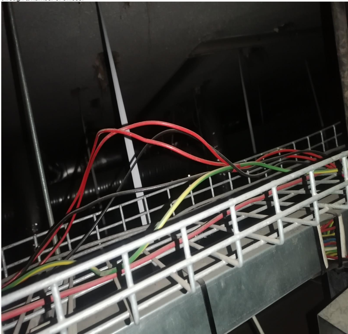
Fig 12 - General Purpose wires running in the cable tray instead of proper enclosed wireway – Cable tray running through a number of offices.
