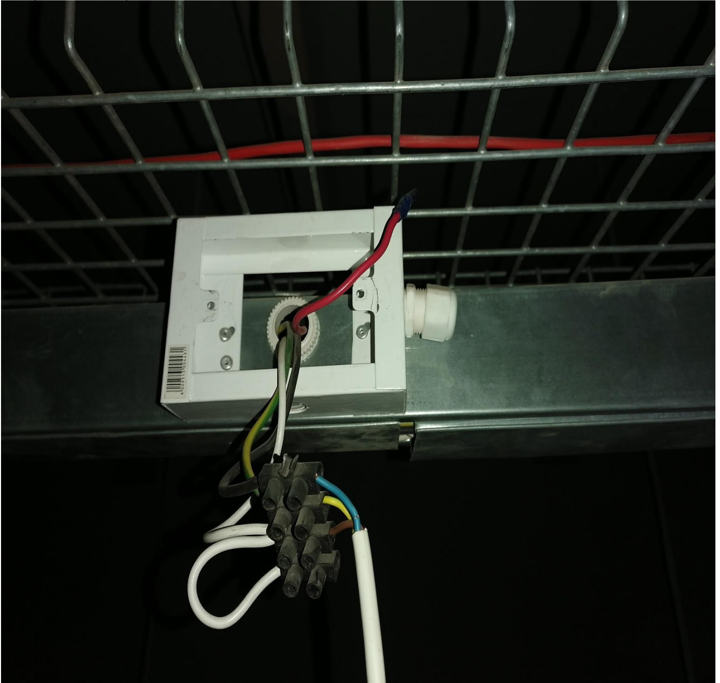
Fig 5 - Open junction boxes exposing connections and improper cable termination (without the use of glands) – Open Plan (Lavika's Office)
