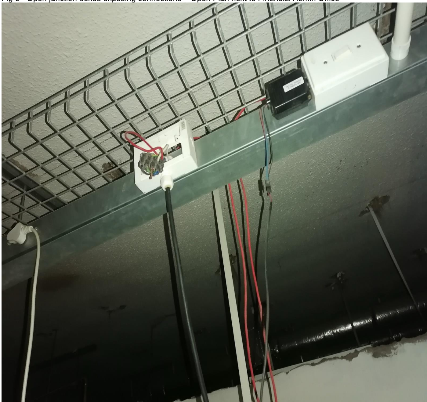
Fig 6 - Open junction boxes exposing connections – Open Plan next to Financial Admin Office
