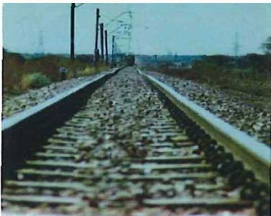
Figure 228: Vertical Alignment Defect Clearly Visible before Tamping
