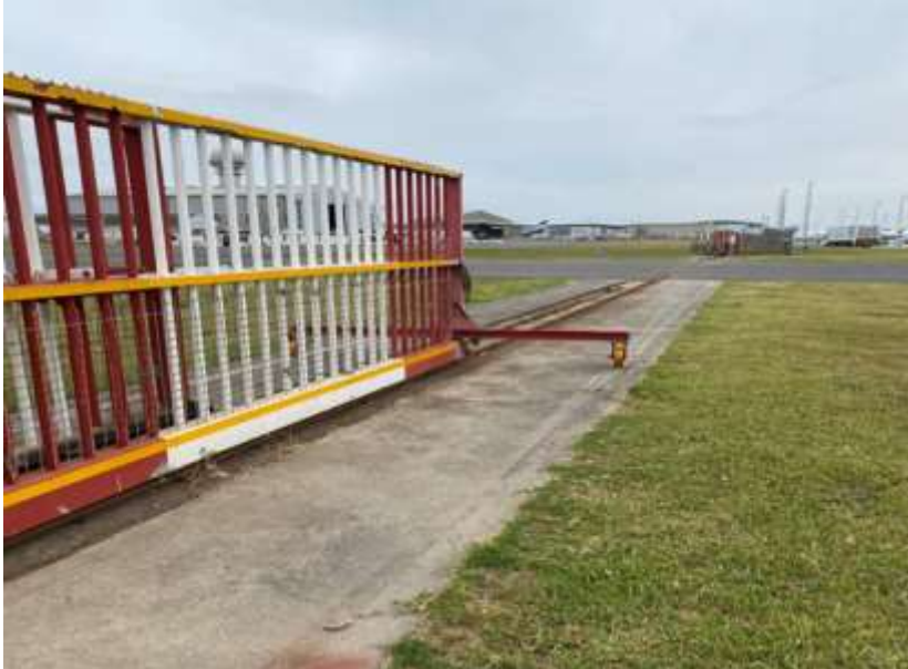
Figure 3.2: Hotel Taxiway Gate at Cape Town International Airport
