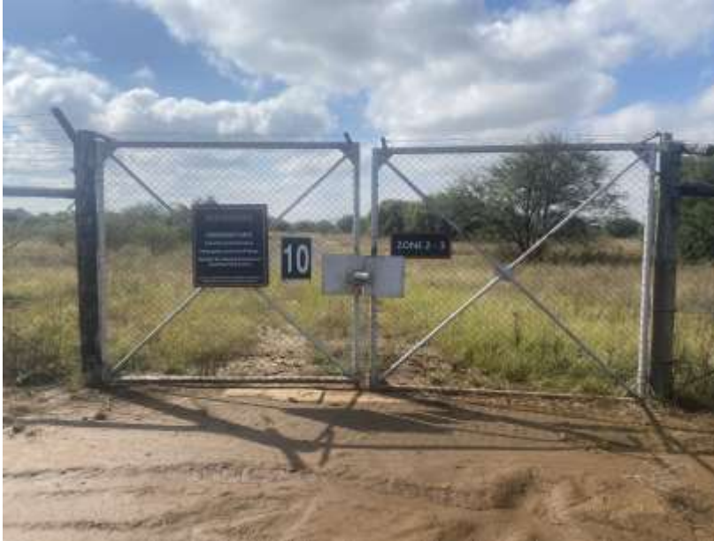
Figure 3.3: Airport Perimeter Gate
