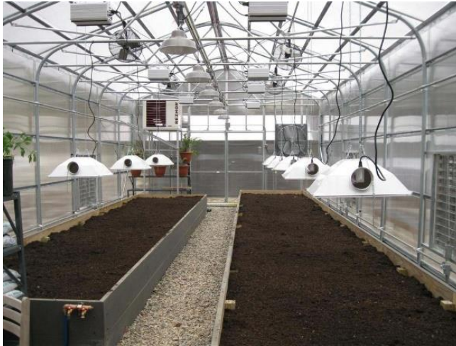
FIGURE 2-8: VAPORPROOF LIGHTING EXAMPLE
