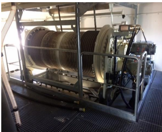
Figure 2(c) Winch house
