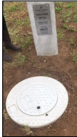
Figure 4 Manhole and marker
