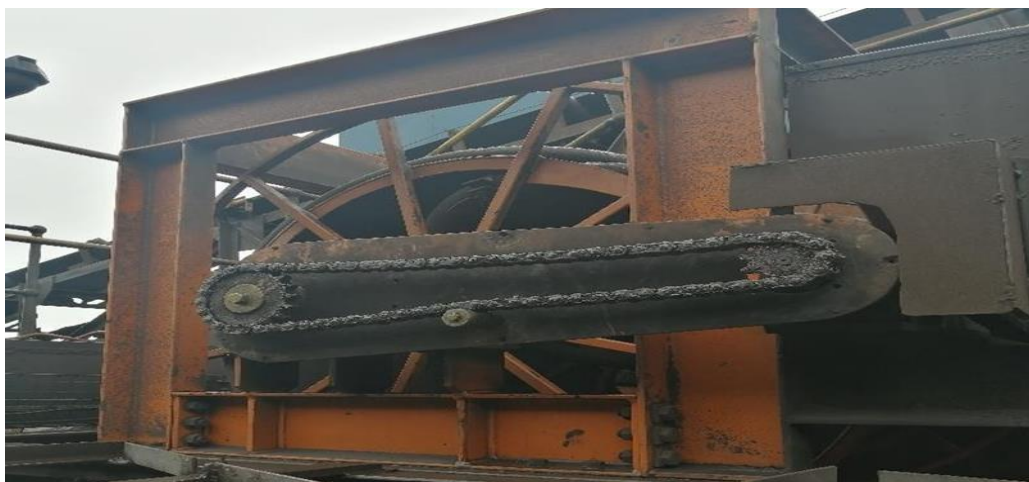
Figure 2: Current Cable Reel Installation
