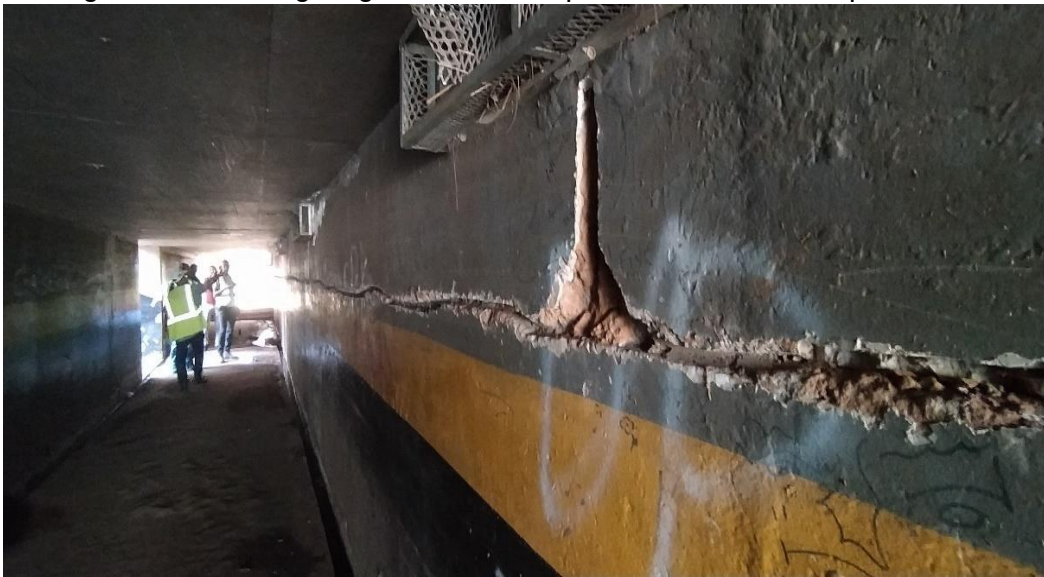
Image 1: Tunnel - Lighting installation required and walls to be painted
