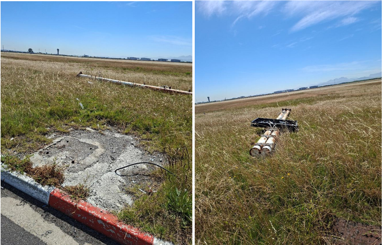
Figure 3.1: Conditions of Concrete base & Steel mast on site
