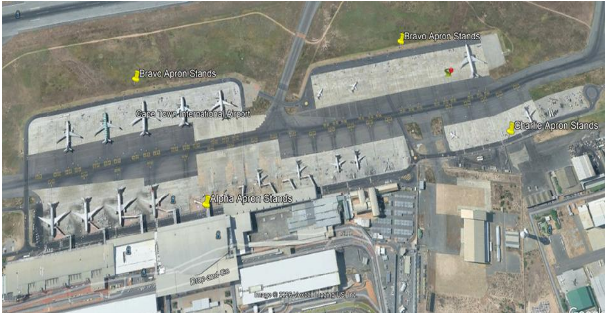
Figure C4.1: Aerial View Image of CTIA Apron Stands
