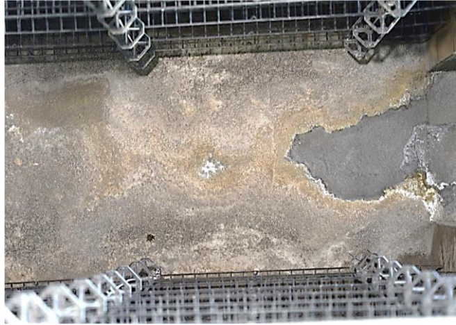
Figure 6: Sulphate Attack
