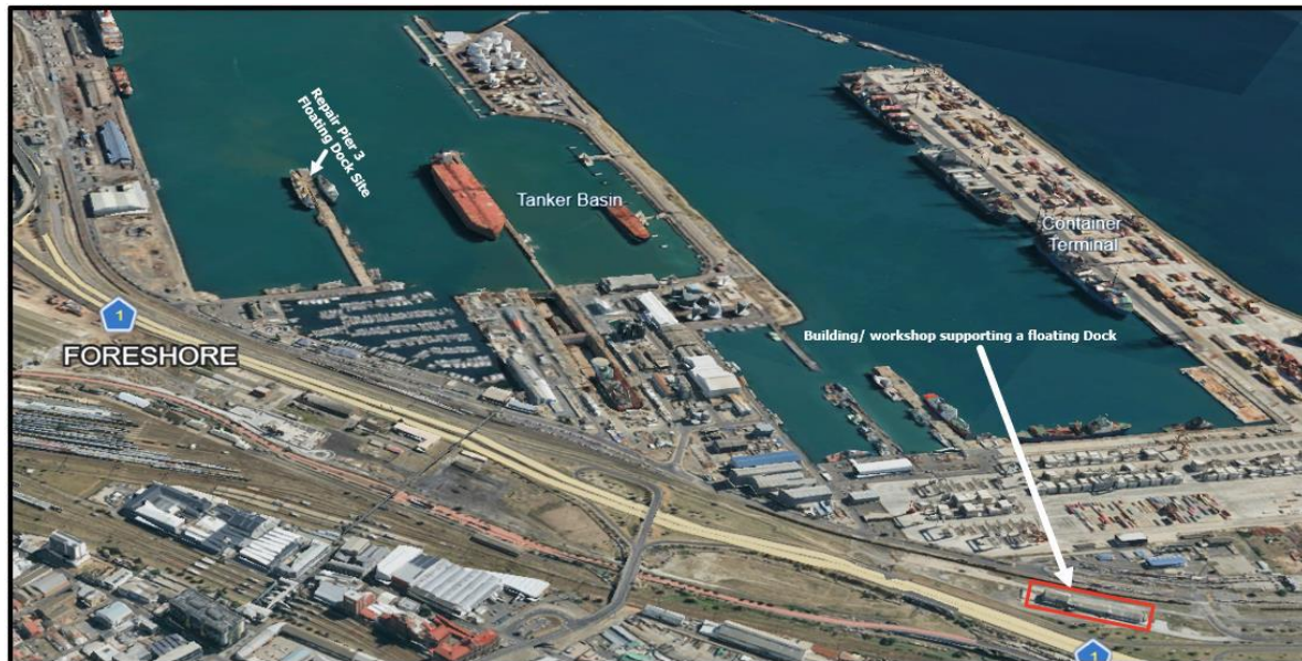
Figure 2: Project Site Aerial View
