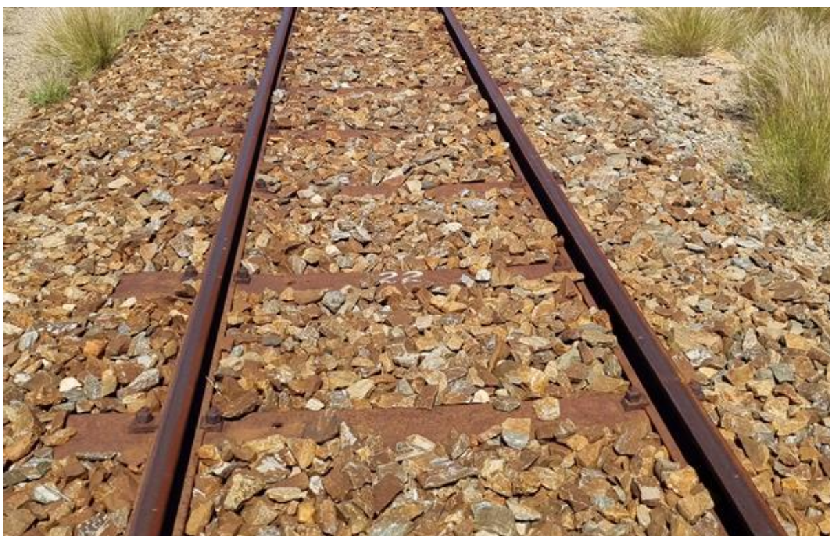
Figure 13: Sleepers and fastenings are intact and in a good condition between km 27 to km 30
