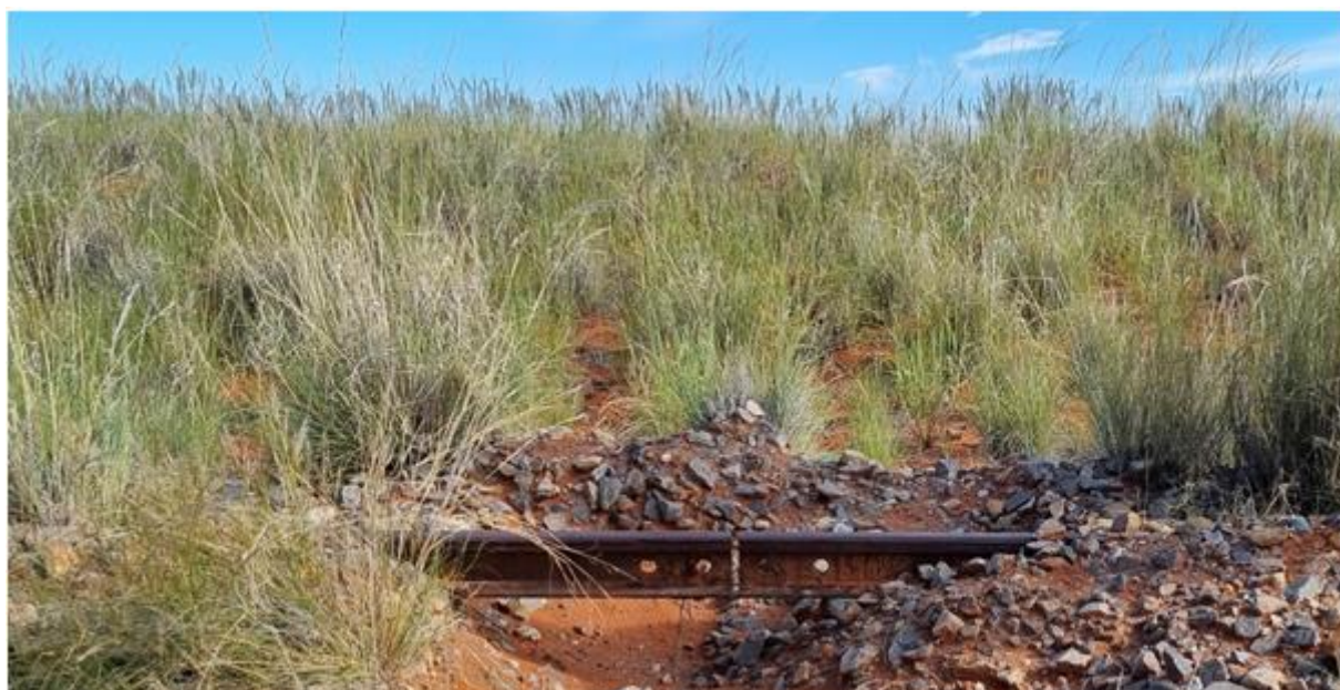
Figure 4: Missing fishplate and bolts at km 7
