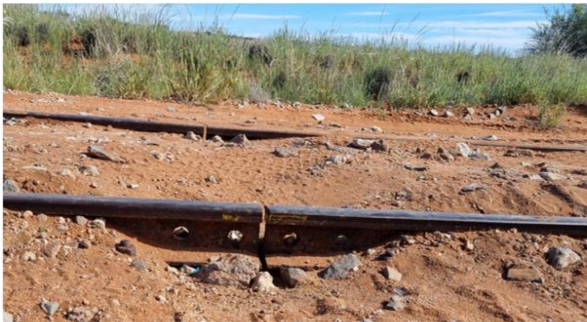
Figure 3: Missing fishplates and bolts at km 4
