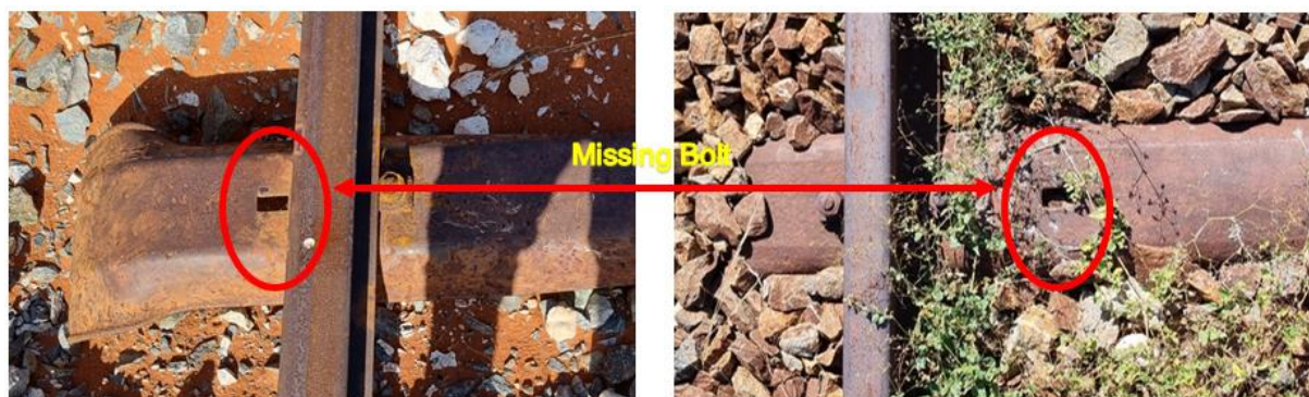
Figure 14: Missing bolts at km 4 and km 26 respectively
