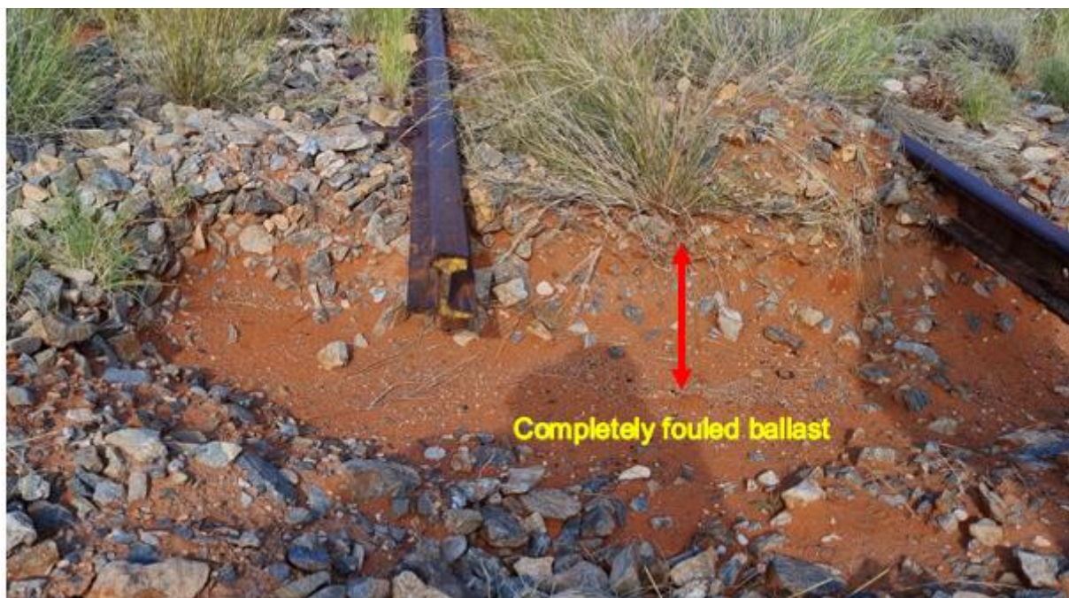
Figure 7: Completely fouled Top ballast layers at km 4
