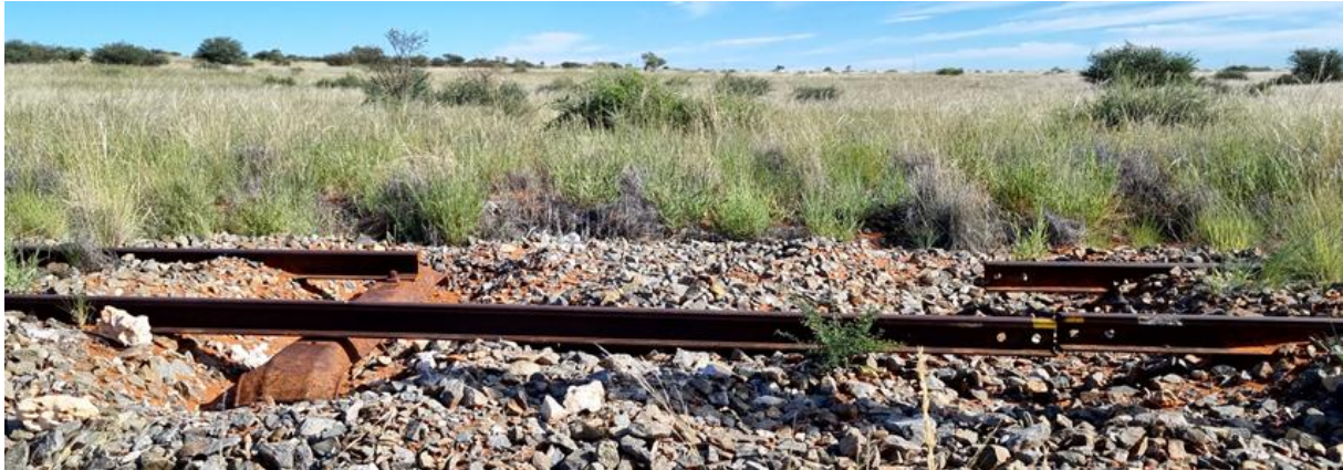
Figure 32: Stolen rails, sleepers and fishplates at km 4
