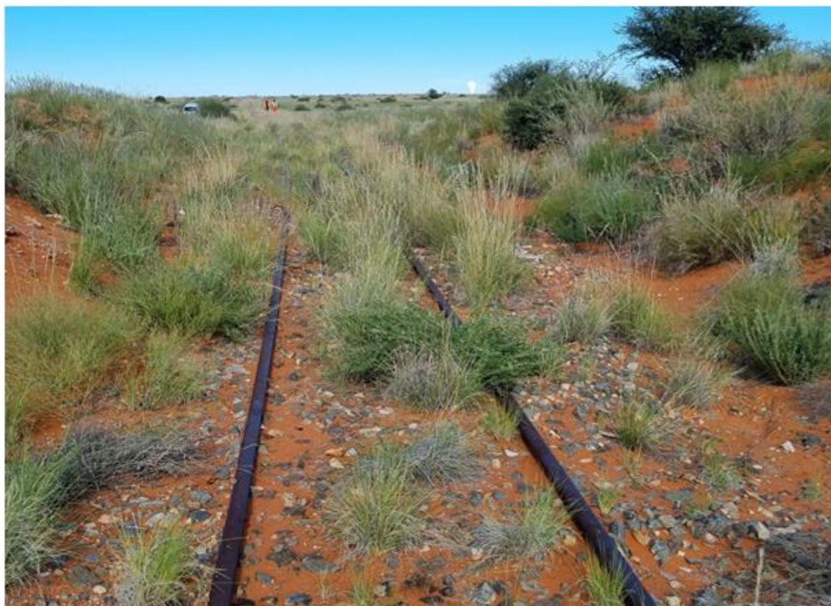
Figure 8: Completely fouled crib and shoulder ballast at km 8
