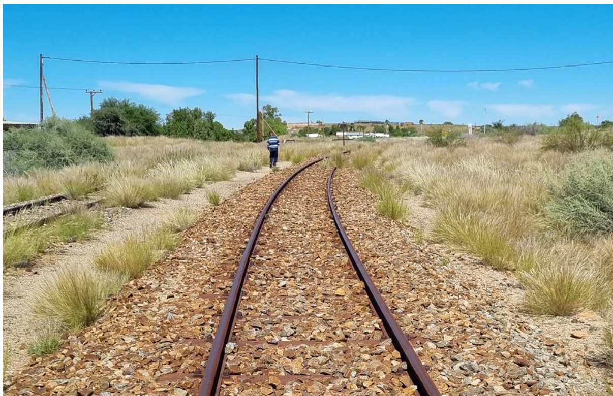
Figure 9: Improved ballast condition but still requiring re-profiling at km 28
