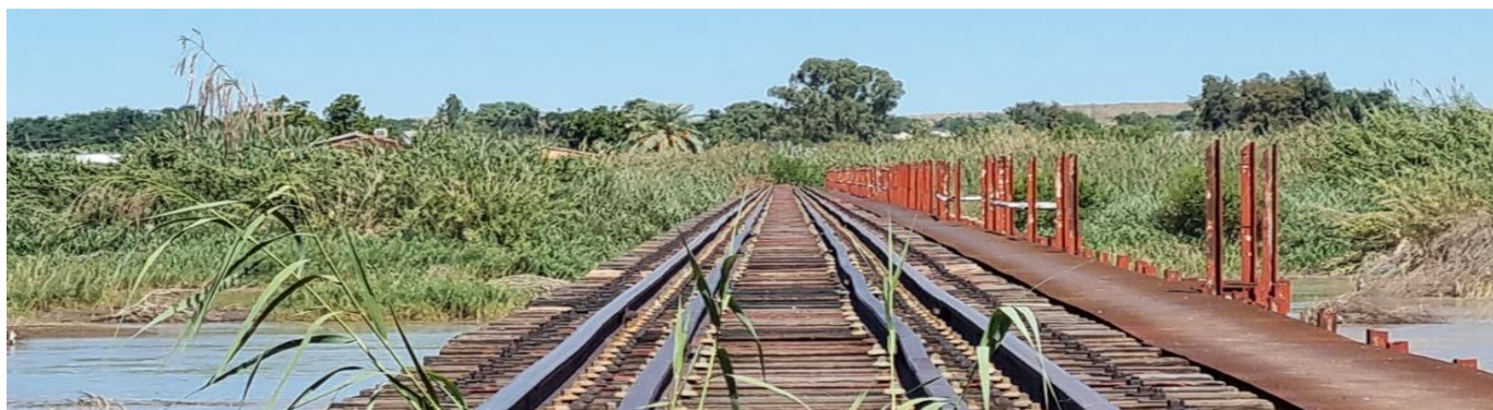
Figure 21: Slacks along the length of the track and missing hand railings on the right
