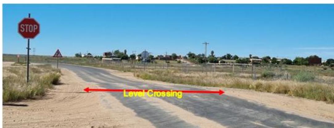
Figure 29: Uneven tar road across track at km 25
