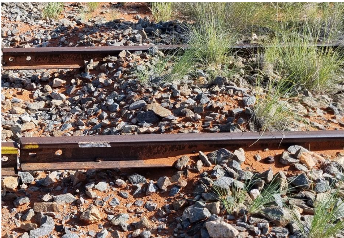
Figure 12: Missing steel sleepers at km 7
