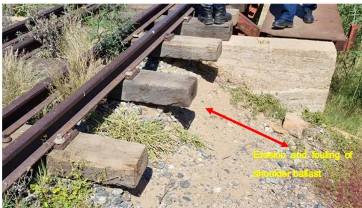
Figure 10: Shoulder ballast erosion and fouling at the Kakamas Bridge Abutment
