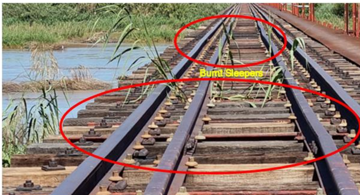
Figure 15: Burnt sleepers on the Kakamas Bridge
