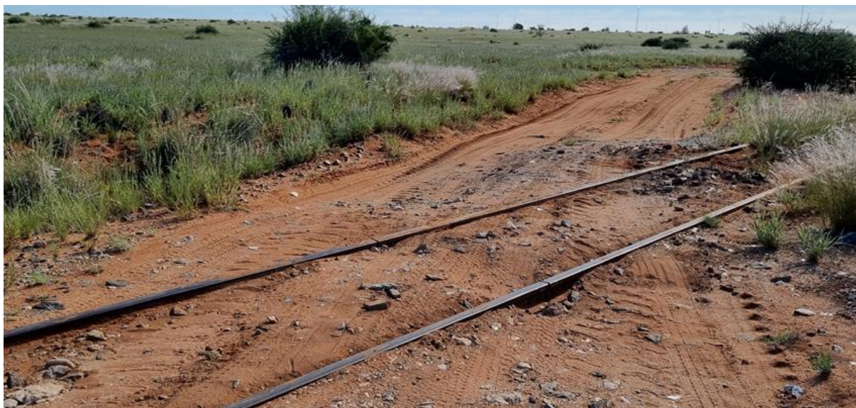
Figure 26: Illegal Level Crossing at km 4
