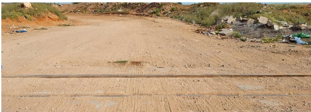
Figure 25: Level Crossing at km 7 covered in sand
