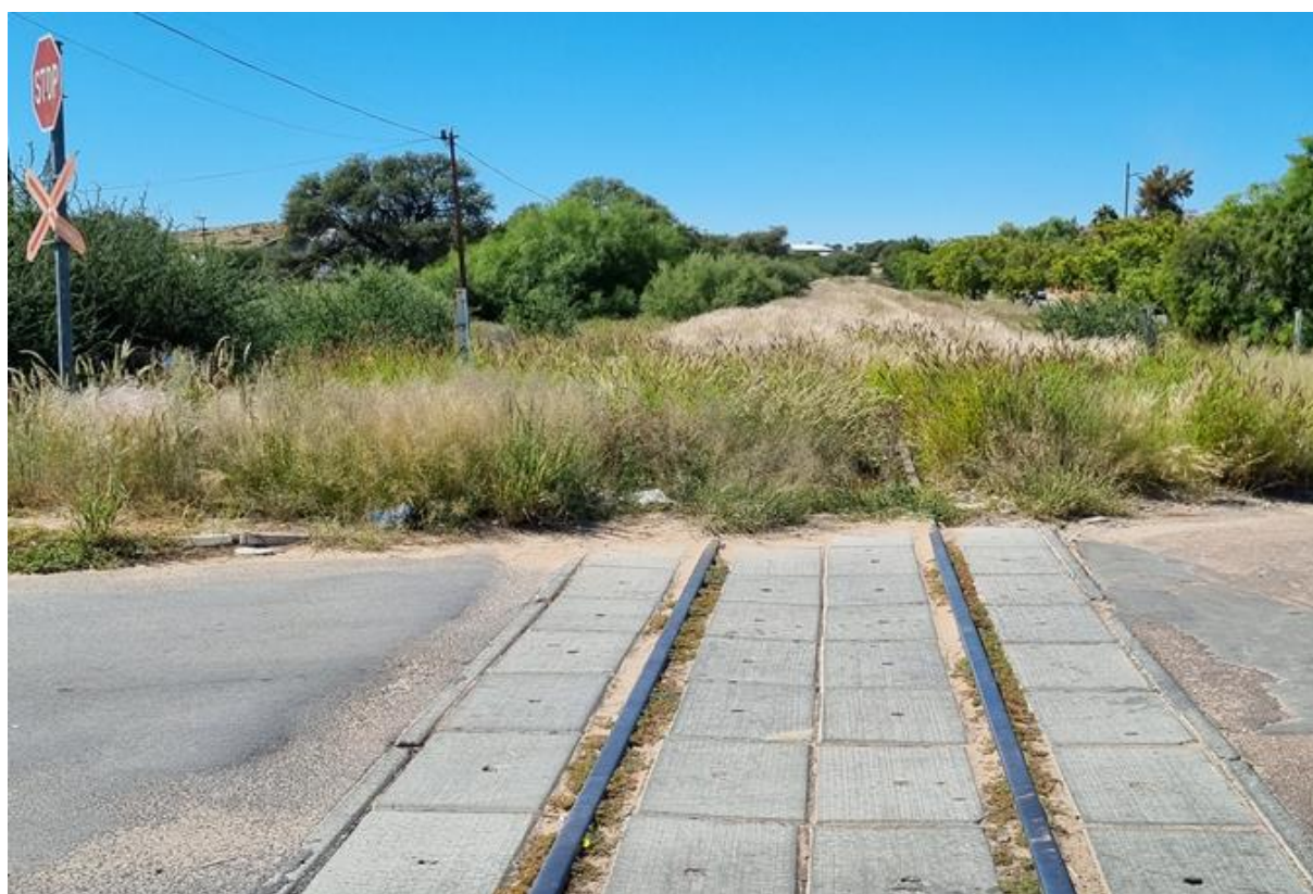
Figure 31: Sand and vegetation between rail and concrete block at the level crossing at km 43
