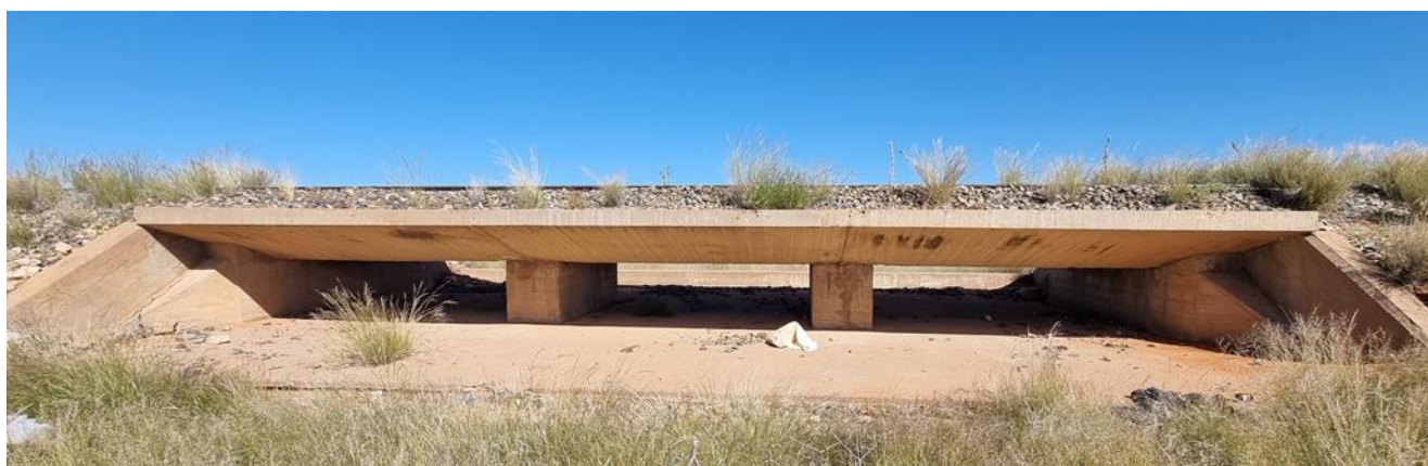
Figure 23: Culvert in good condition at km 13
