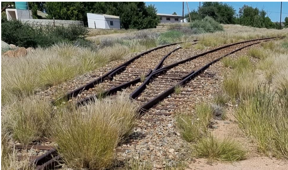
Figure 19: Turnout at Geelkop in good condition, with over grown vegetation
