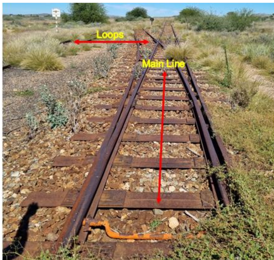
Figure 17: Turnout at Kanoneilandweg in good condition, with over grown vegetation
