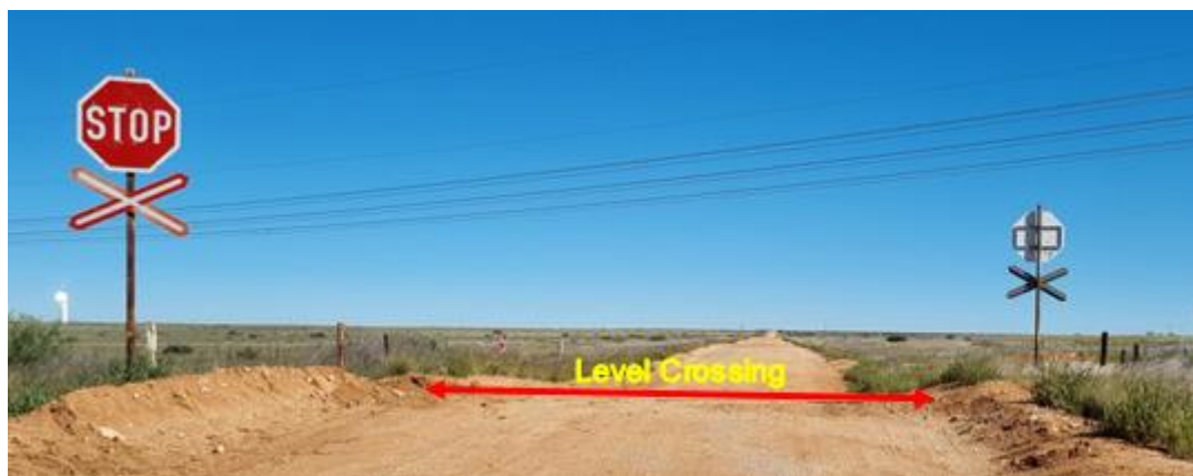
Figure 28: Graded road covering the track and excess material obstructing the line at km 22
