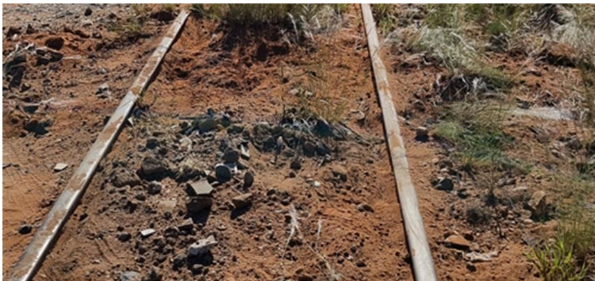
Figure 11: Sleepers fully submerge in sand at km 4
