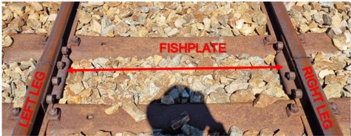
Figure 5: Fishplates on both legs at km 28/ km 29 (between Kanoneilandweg and Geelkop)
