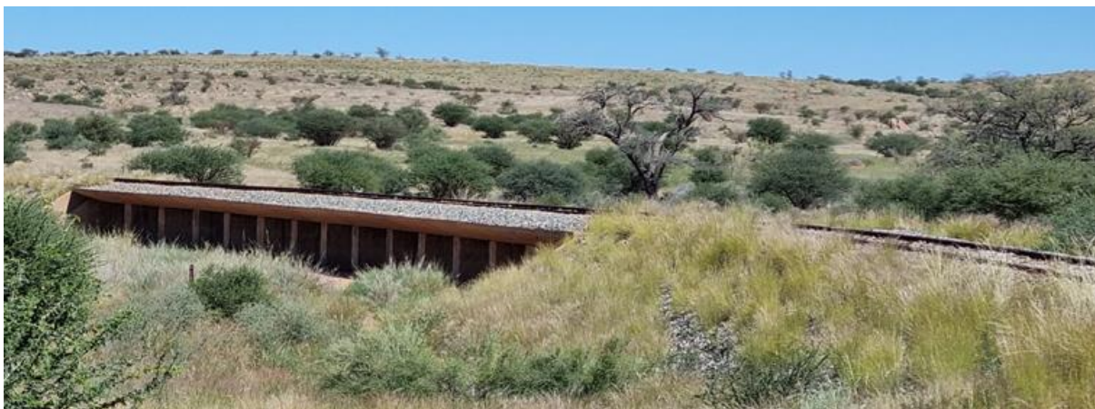
Figure 24: Culvert between Geelkop and Keimoes appears to be in a good condition
