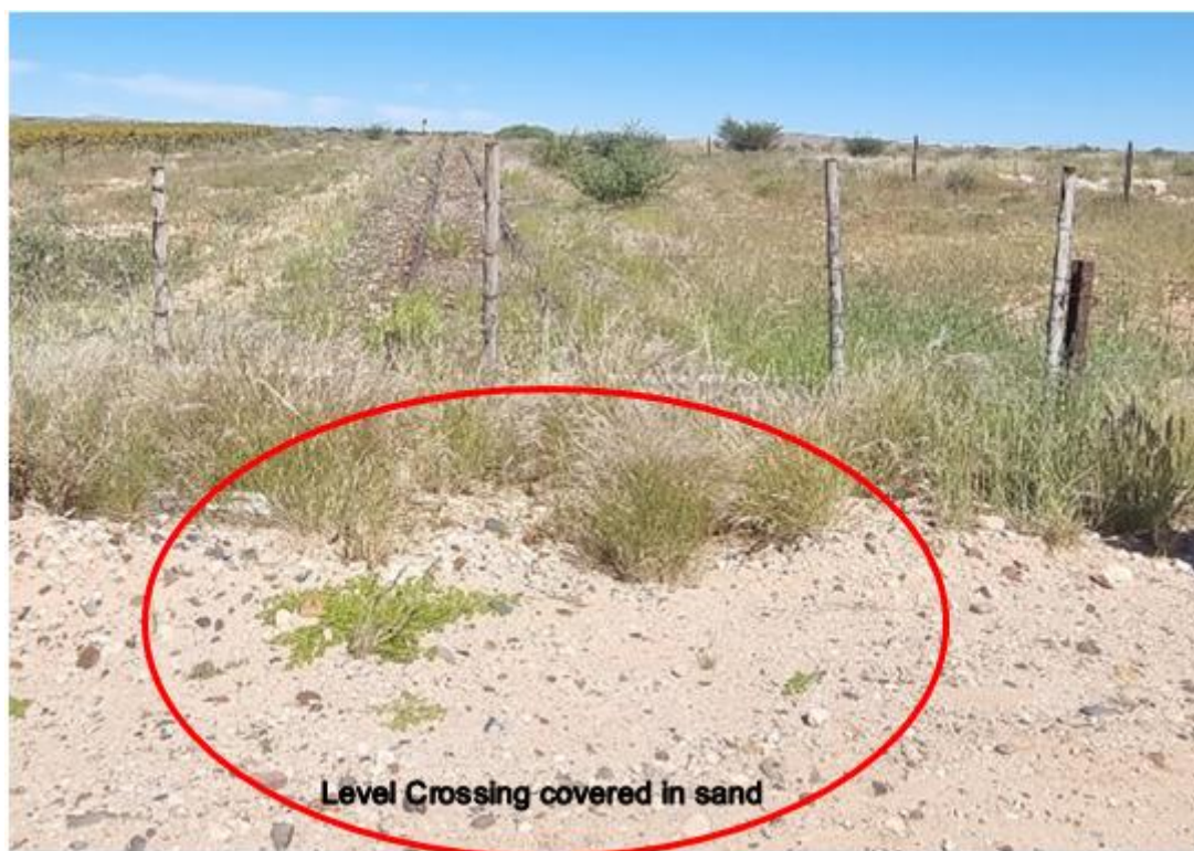
Figure 30: A gate build on track and track covered in sand at level crossing at km 27
