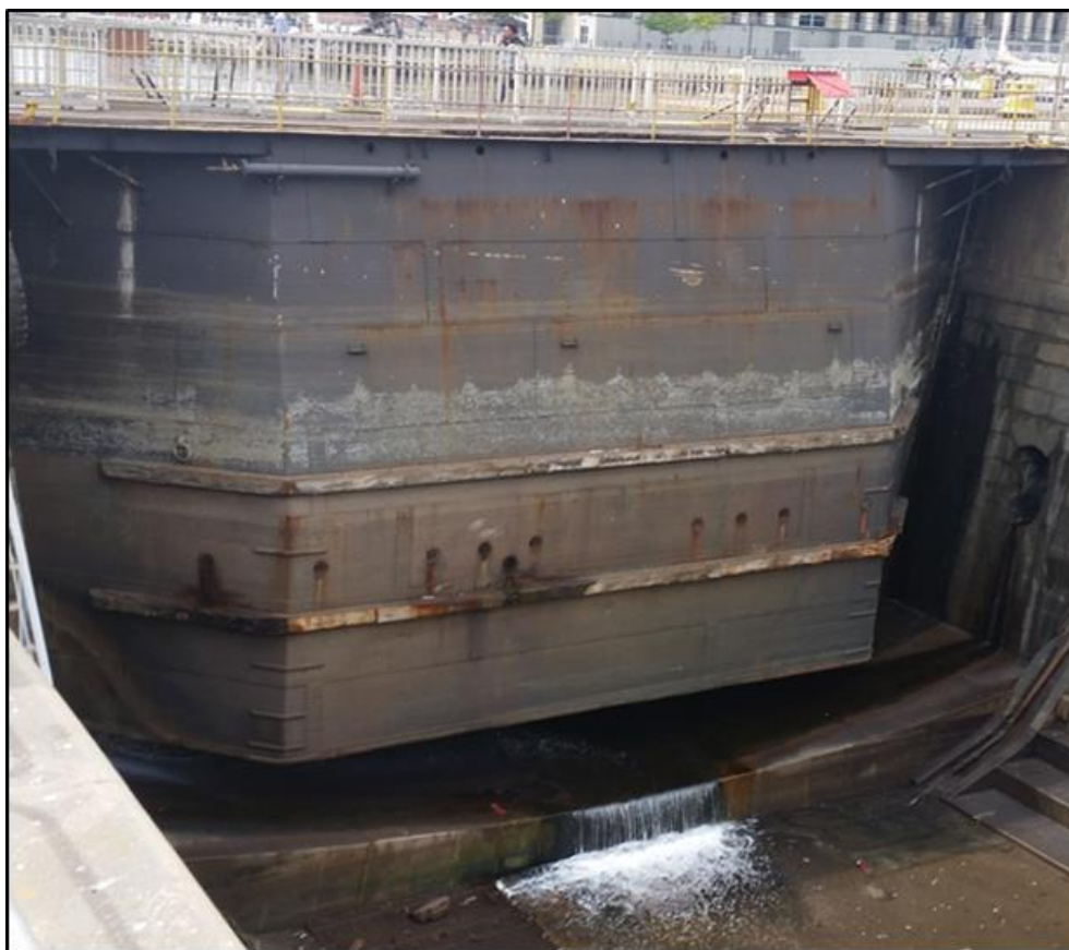
Figure 1: Floating Caisson in operational position
