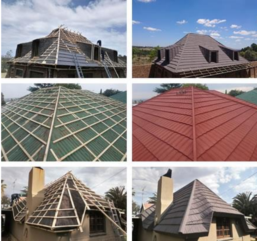
Figure 6 CORRUGATED ROOF TO BE REPLACED WITH HARVEY TILES (EXISTING ROOF NOT TO BE REMOVED)
