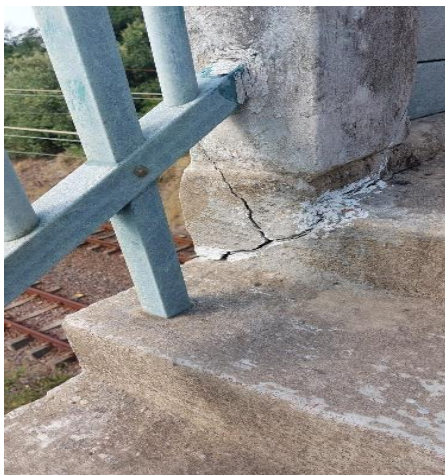
Figure 4: Concrete Bridges Flaking Concrete panels
