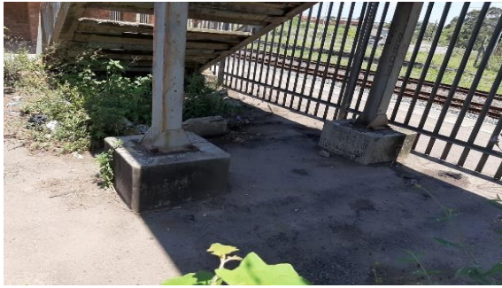
Figure 2 Missing Bracings on Columns bracing
