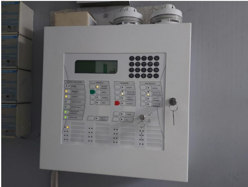
Fire Main Panel at ACSA Rest room and Fire station.
