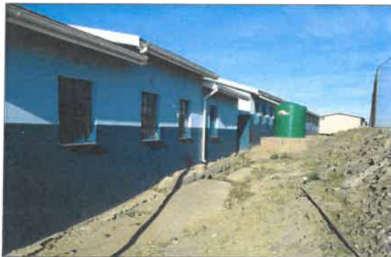
Picture 1: The existing classrooms located east and downslope of the existing netball court
