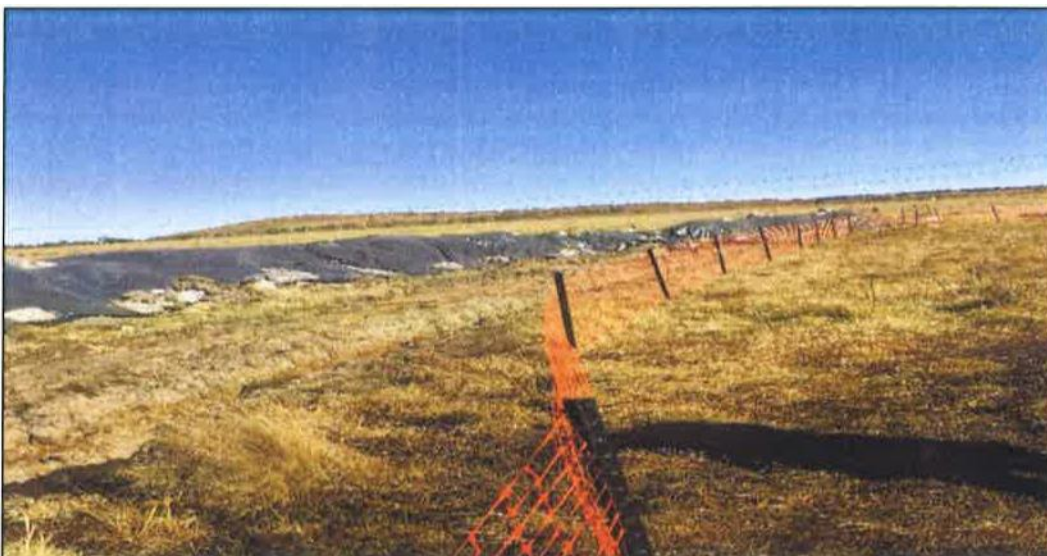
Figure 2: Snow net fencing on site.
