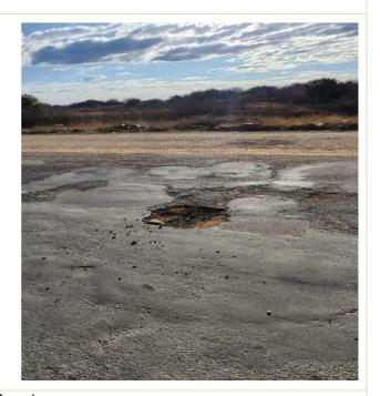
The photos shows that potholes are forming on the surfaced area
