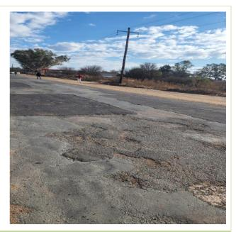
The photos show the base is left exposed to natural element that can cause pavement failure. General disintegration of total asphalt layer.
