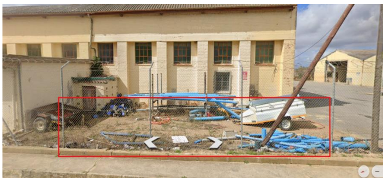
Area where paving is to be placed
