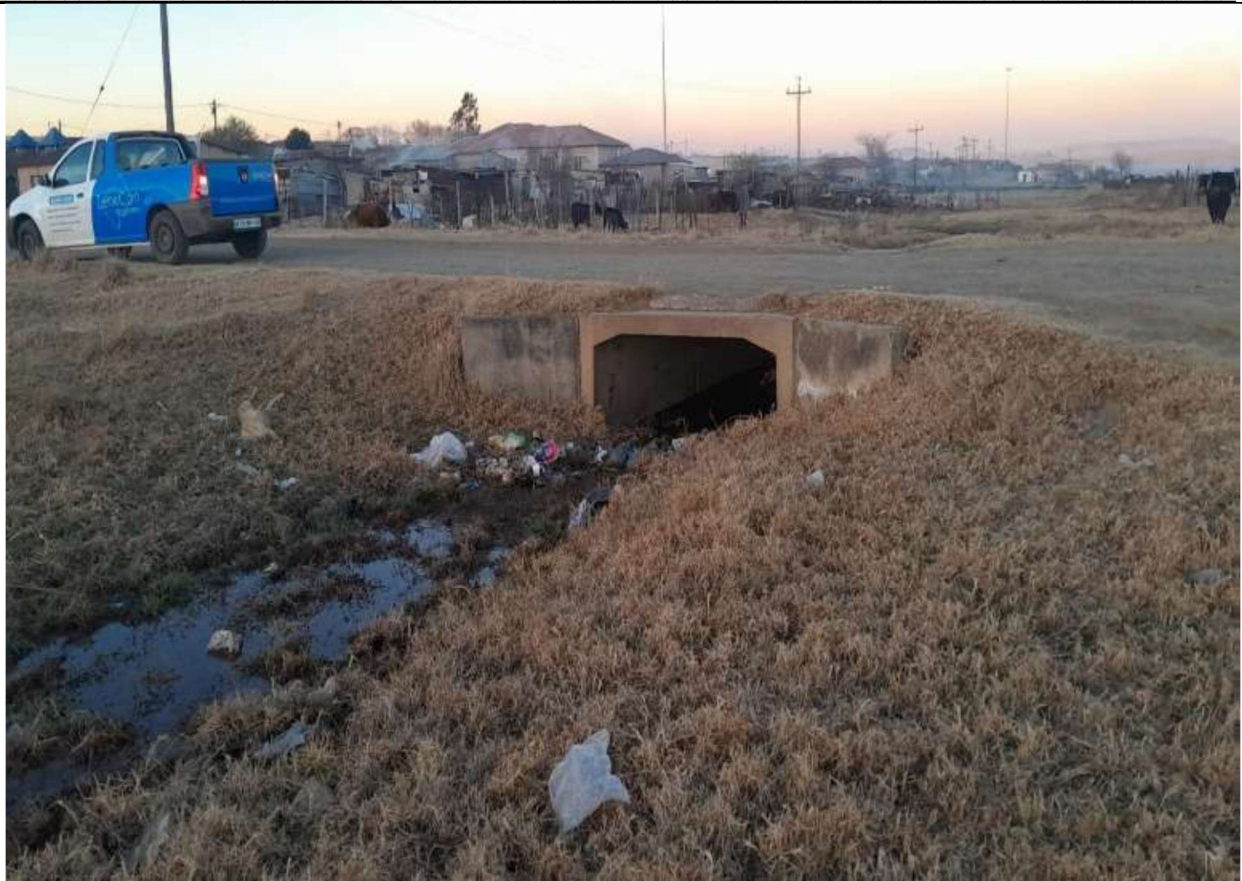
Existing culvert crossing
