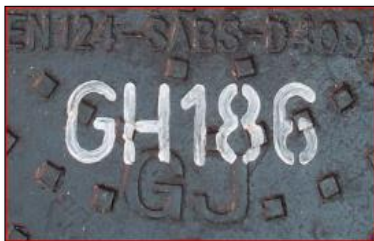
Fig. 25 Manhole number painted on cover
