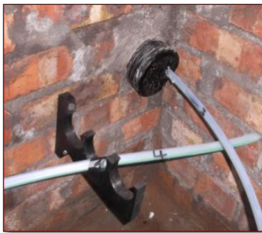
Fig. 23 Brackets and duct spacing (example)
