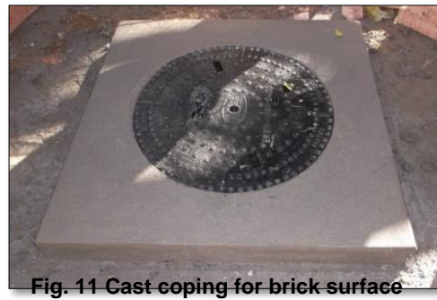
Fig. 11 Cast coping for brick surface
