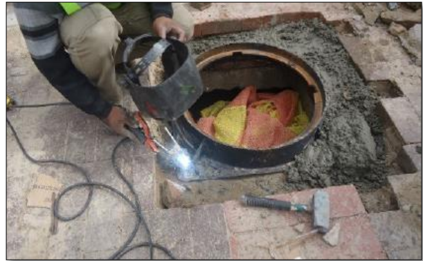
Fig. 17 Welding the frame in place
