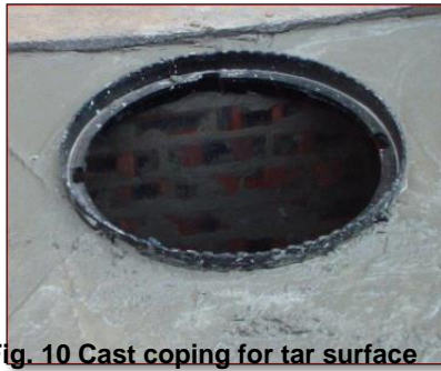
Fig. 10 Cast coping for tar surface
