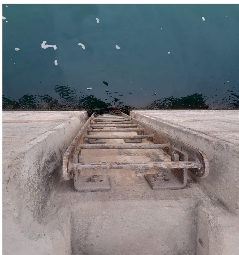
Figure 1 (corroded Access quay ladders)
