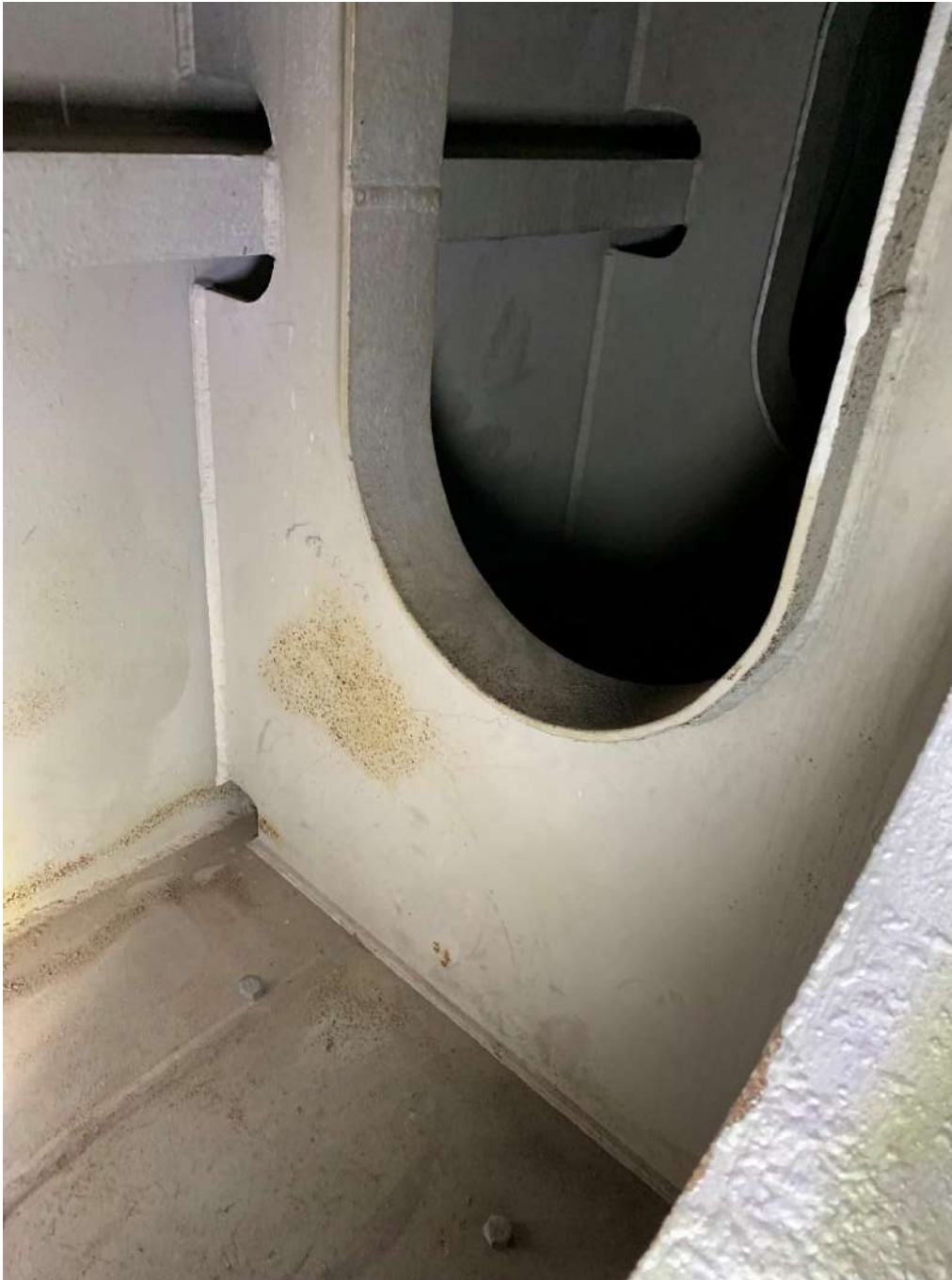
Photo 5 Tippler Rail Platform Internal Surface Corrosion
