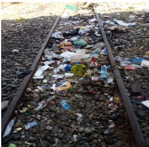
The sleepers not visible and covered by the garbage at Limindlela
