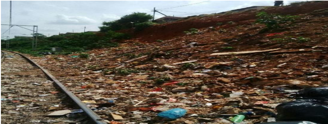
The sleepers not visible and covered by the garbage at Limindlela
