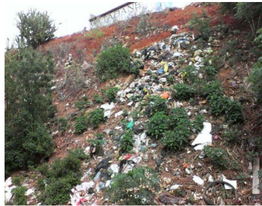
The garbage on the embankment at Limindlela
