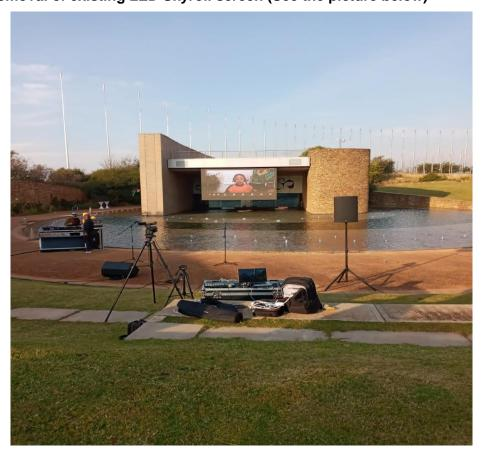
The above screen was bought and installed in 2010. The LED screen is currently faulty and non-functional. The screen is mounted right on top of the roof slab of the Sanctuary building facing towards the Eternal flame and Amphitheater. Those are the two elements of the Freedom Park which must be taken care of when installing the new screen as they must always be visible.
