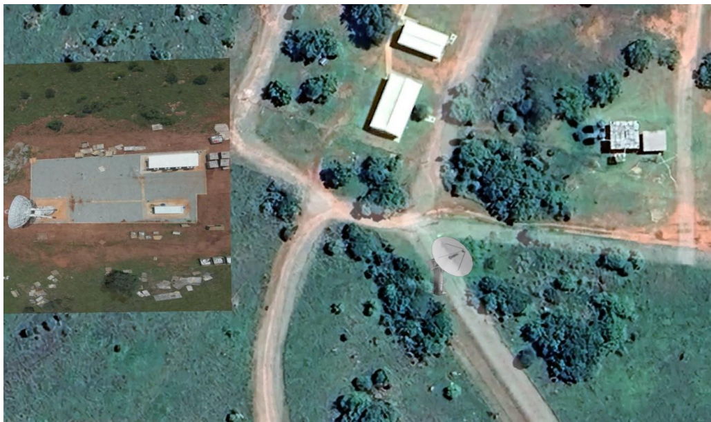
Figure 2: S, X, Ka Antenna Location
