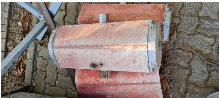
6. Replace 12 x pneumatic actuators – Air scour valves
