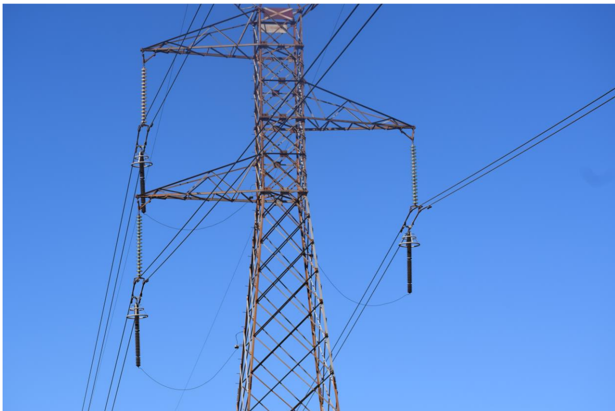
Fig 1: Typical Installation of LSA's on Hera-Watershed 275kV Line.
