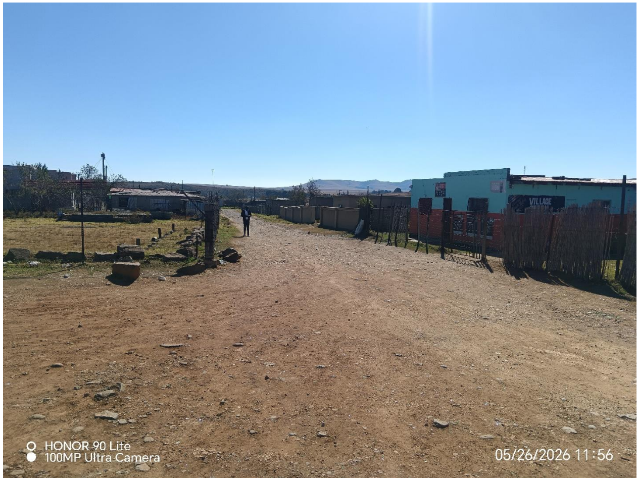
Start of road 2
