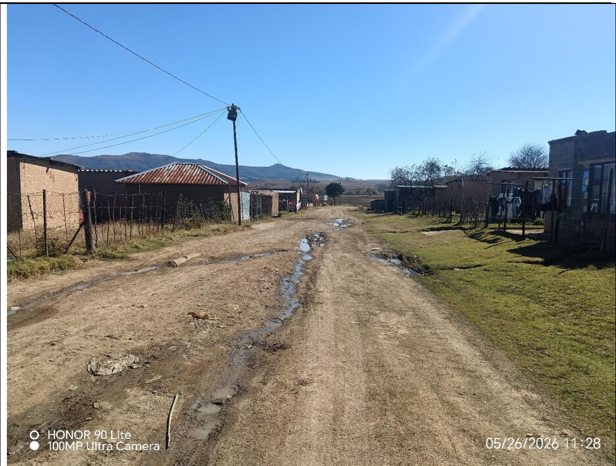
Road 1 Ward 5: Flowing water from household taps
